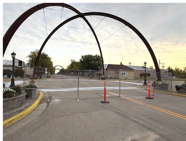
Coco paving was contracted by the RM of Russell-Binscarth to replace the crumbling crosswalks on Main Street. A total of 16 crosswalks at 4 intersections were replaced with concrete, providing a much-needed repair for pedestrians and drivers too!
